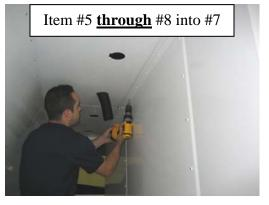
Pre-drill through **Ceiling** sections, (using **Divider** as a template), with 3/16" drill bit and attach using ½" x 1 ½" hex head lag bolts
